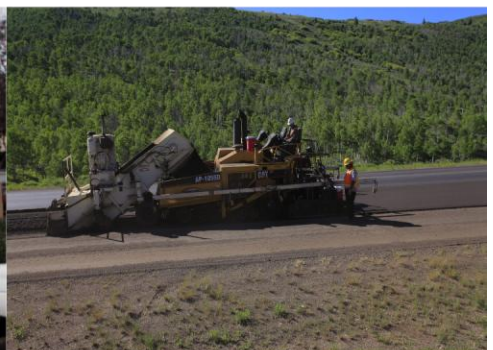
9. OVERLAY WITH NEW HMA SURFACE
