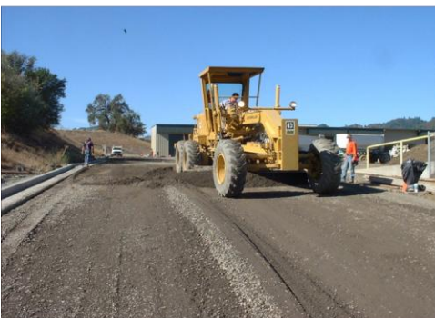
7. FINISH GRADE IN PREPERATION FOR NEW HMA
