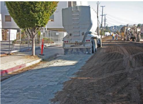
4. DISTRIBUTE CEMENT OVER RECYCLED MATERIAL
