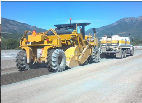
5. HYDRATE CEMENT AND BLEND WITH RECYCLED BASE
