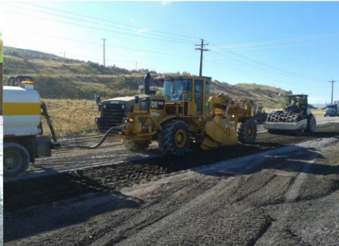
2. PULVERIZE DETERIORATED ASPHALT AND ROAD BASE
